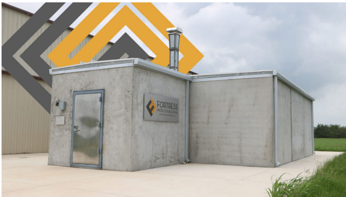
FIGURE 2 A FORTRESS protective building utilized as an MRB for operators. 9
